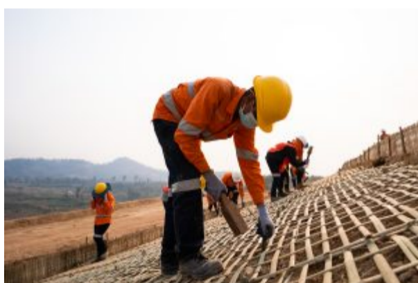
ກິດຈະກຳພື້ນຟູ – ປູກະແຕະໄມ້ໄຜ່ດັກຕະກອນ/Rehabilitation activity – bamboo matting
